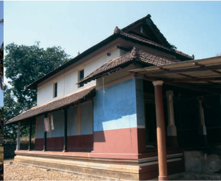
Plate 4: The widely projecting roofs are held up by pillars from below, creating laterally open but shaded ambulatory paths, bordered by thick mud walls as here at Padangady
