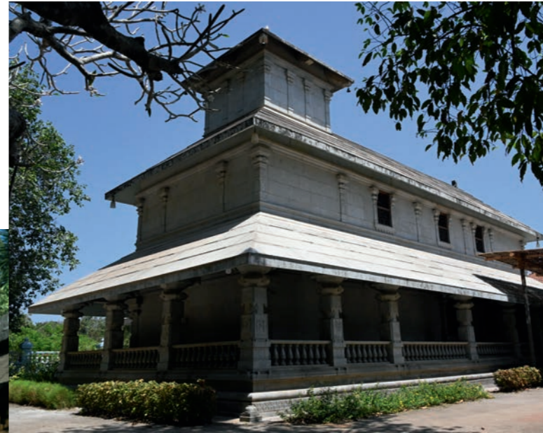
Plate 8: Although the Candranatha Basadi at Dharmasthala is a contemporary concrete structure, it follows the traditional style of having projecting tiered roofs and an open arcade.
