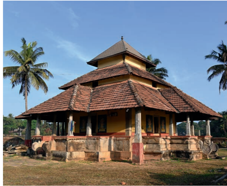
Plate 2: The Kere Basadi at Karkal is typical of the regional Jaina temple architecture by having multiple slanting, tiered roof structures.
