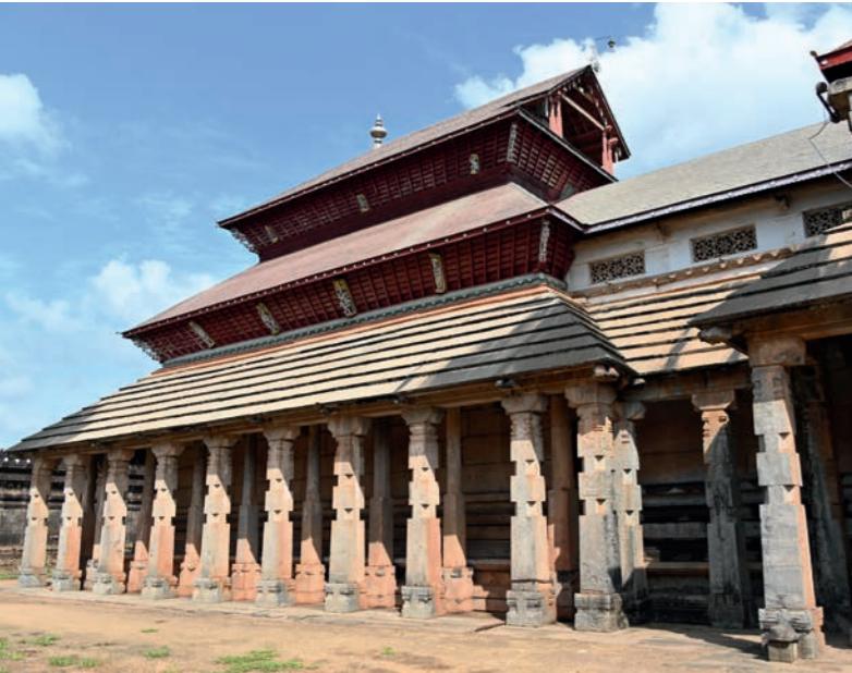
Plate 6: While the lowest roof level of the Candranatha Basadi at Mudabidri has been made of hard stone, the upper tiers show combinations of wood, tiles and copper sheeting.
