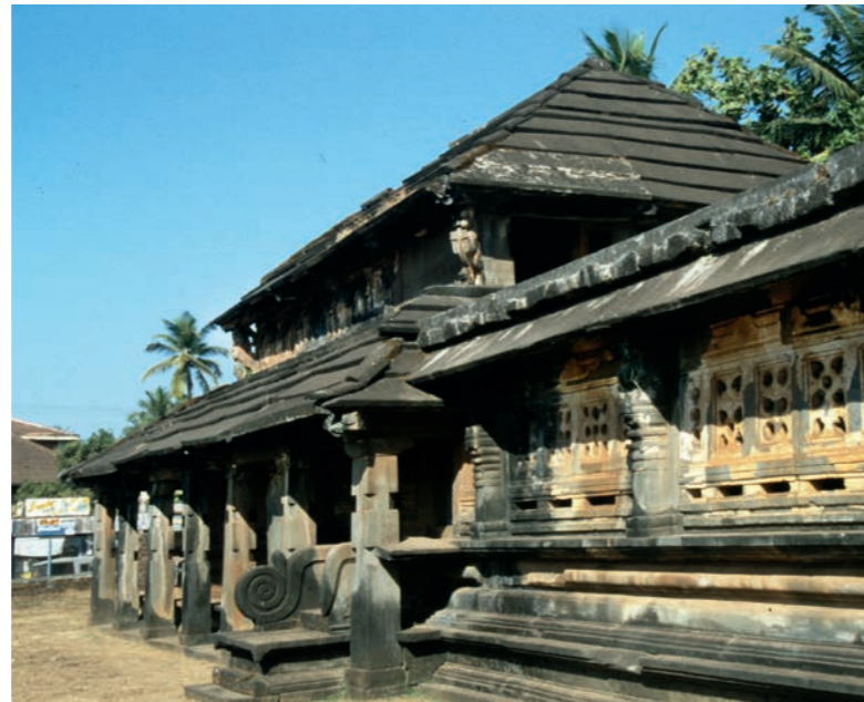
Plate 7: The Chandranateshvara Basadi at Bhatkal was built entirely of imported stone, including both of its tiered roof structures
